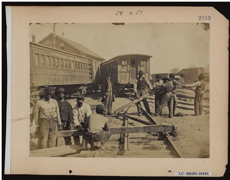
[Military railroad operations in northern Virginia: men using levers for loosening rails] 4
